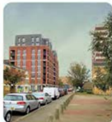
Completed High Path Phase 1
