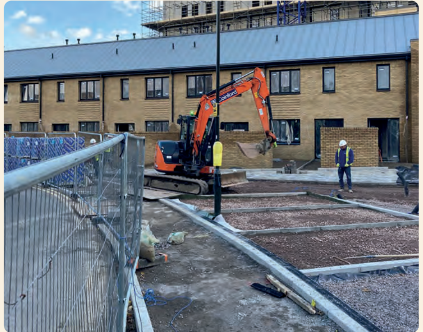
The mews houses along Rodney Place
